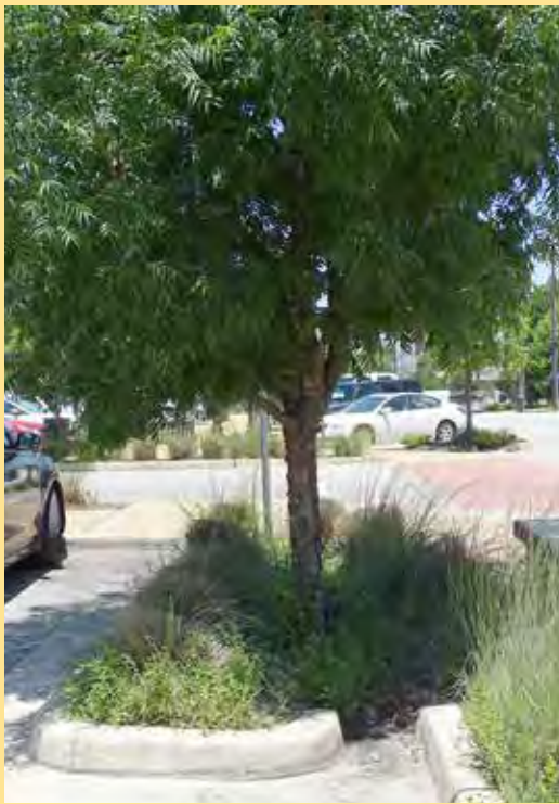
This tree in a bioswale is green infrastructure because it is part of a stormwater best management practice (BMP).
