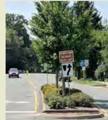
Streets were narrowed with new tree islands and bump outs with trees were added to sidewalks to shield pedestrians and slow traffic.
