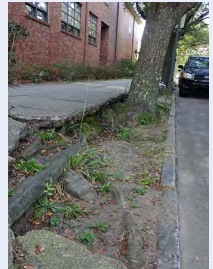
It’s not the tree’s fault that this planting area was never large enough for this tree.
